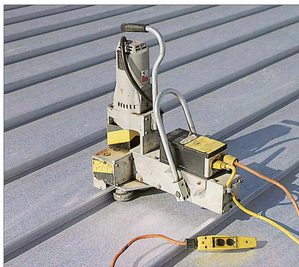
6 Roof panels overlap and are sealed together with a mechanical seamer.
