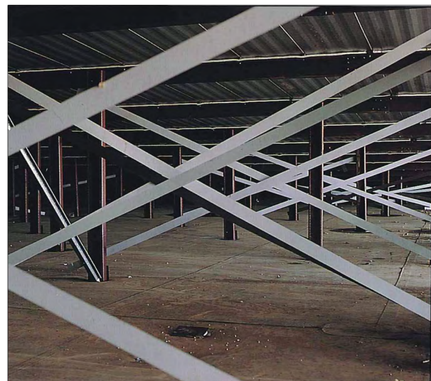
4 Cross bracing reinforces the completed framing.
